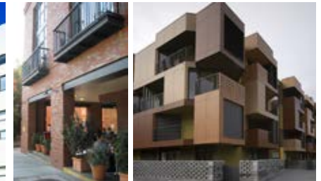
Building line variation
